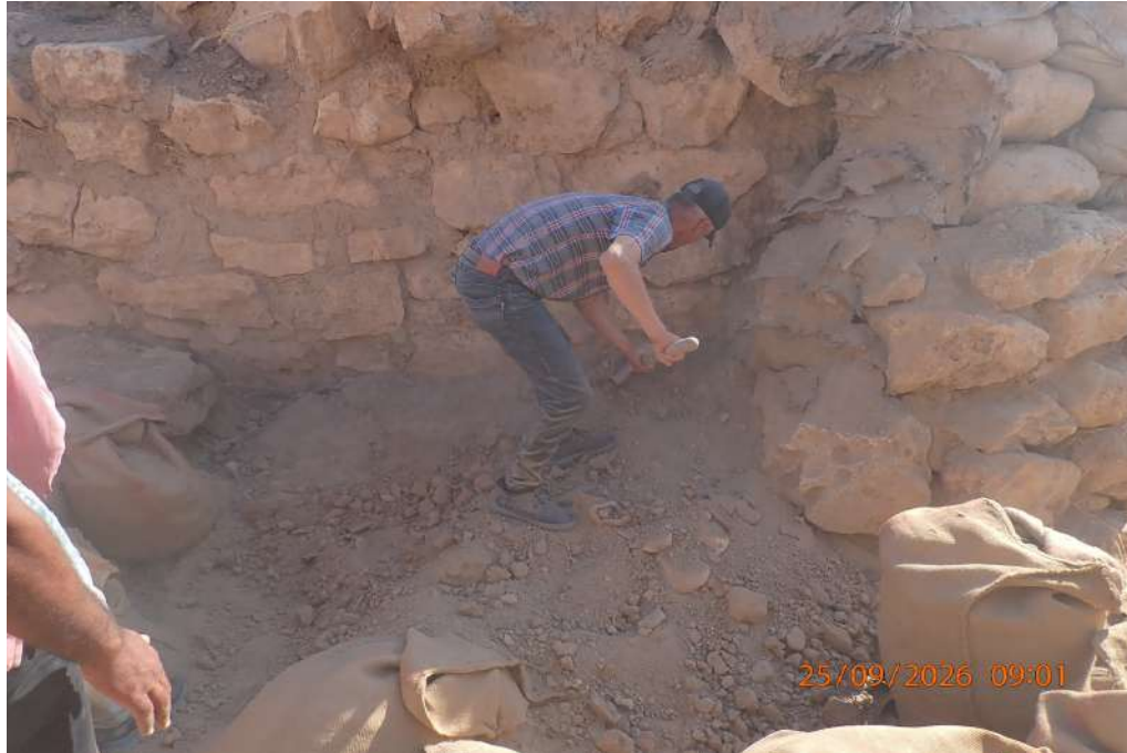
Fig. 5: Levelling the ground before placing the sandbags.
