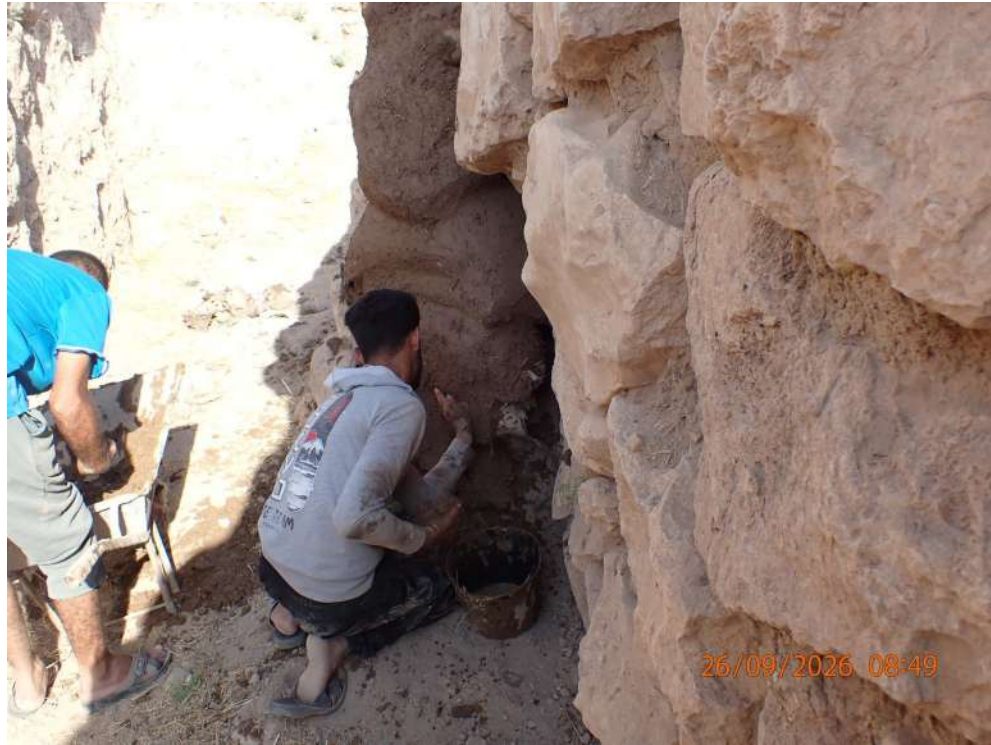
Fig. 11: Plastering the right-hand side
