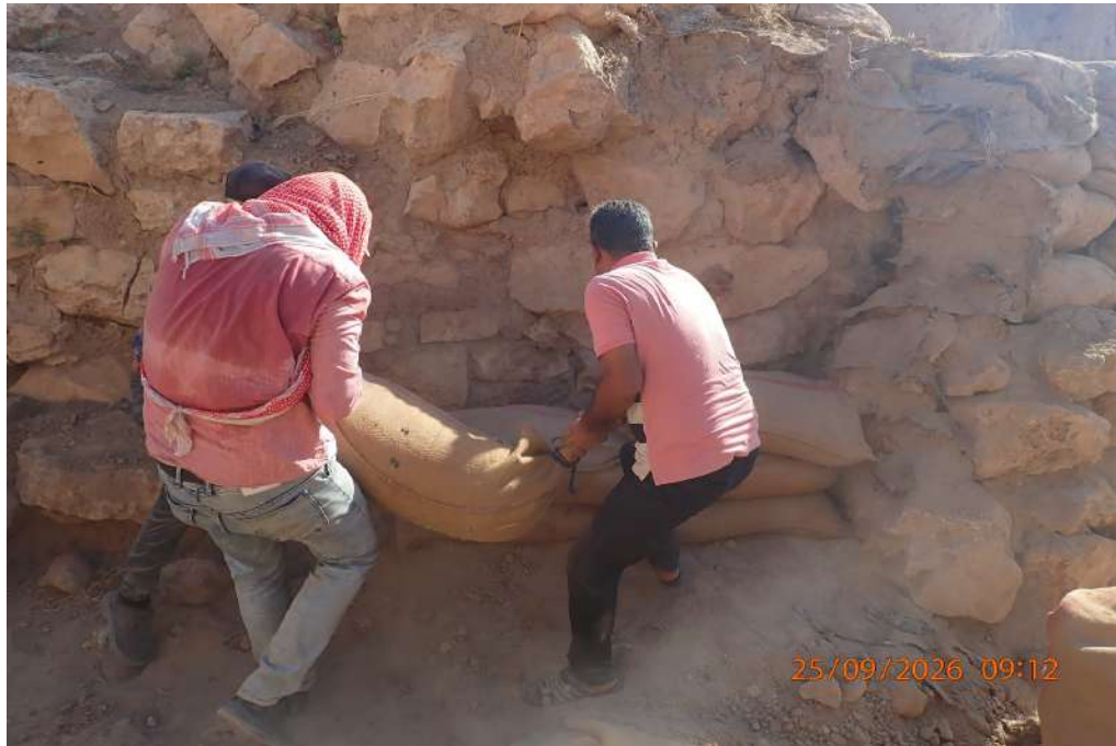
Fig. 7: Placing the sandbags on top of one another.
