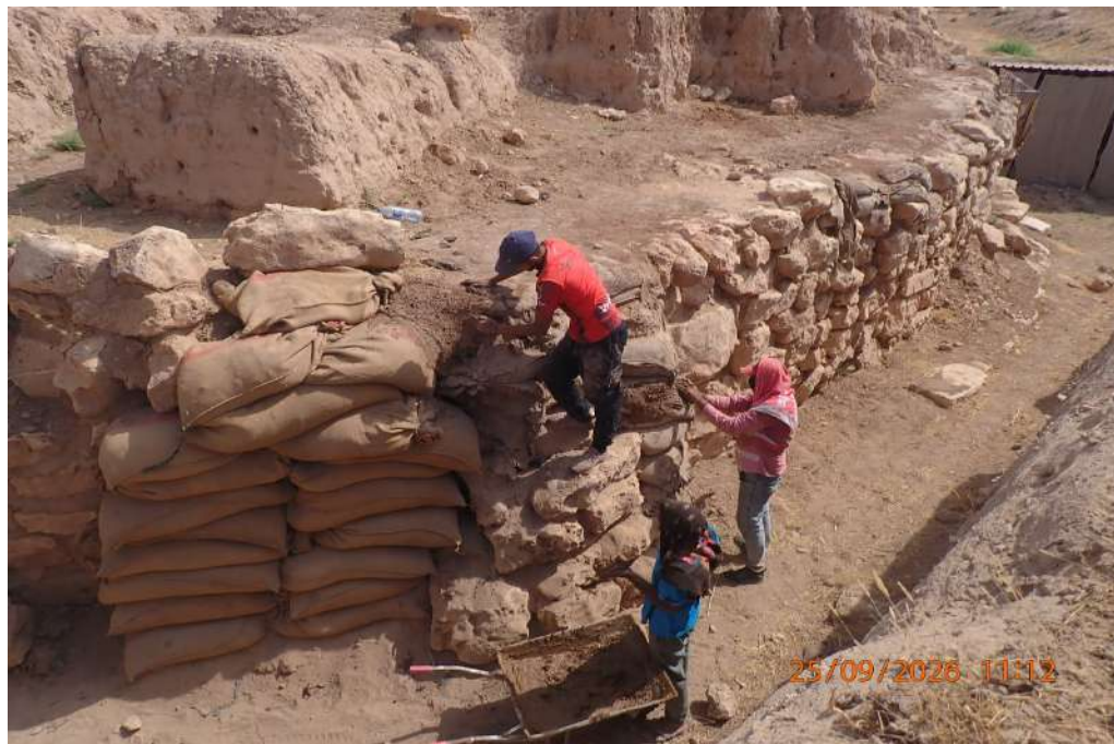
Fig. 10: Plastering the upper levels of the wall
