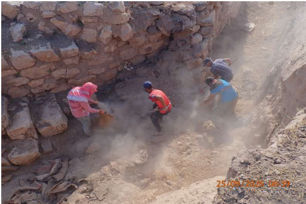
Fig. 6: Filling the sandbags with soil.
