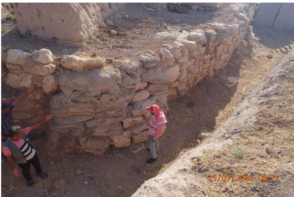
Fig. 2: General view of the retaining wall before the intervention.
