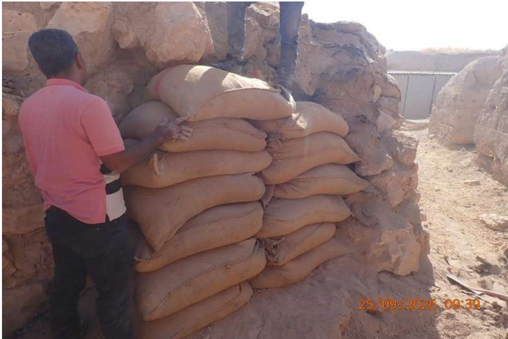
Fig. 9: Placing a sandbag beneath the stone.
