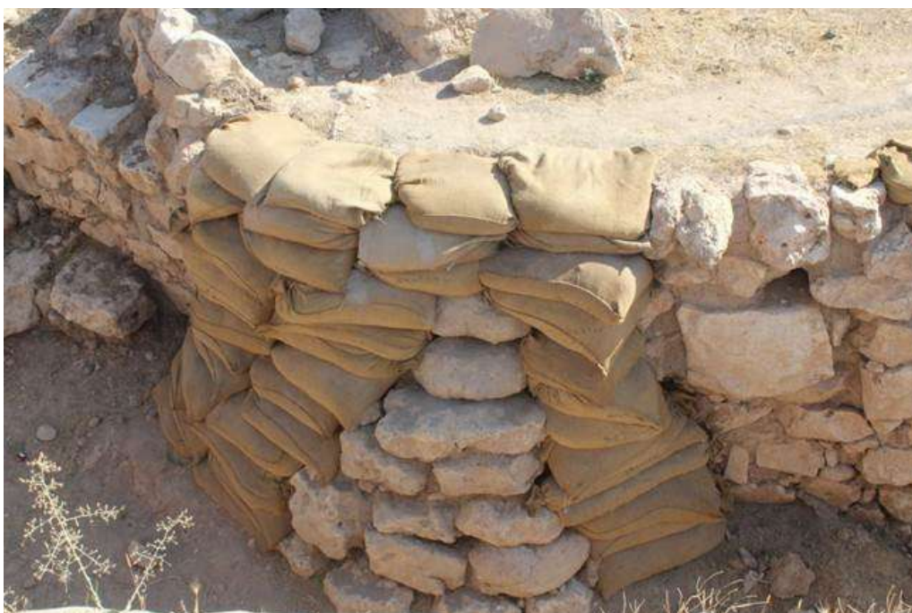
Fig. 1: General view of the retaining wall in 2019.
